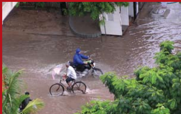
Flooded Road, India
